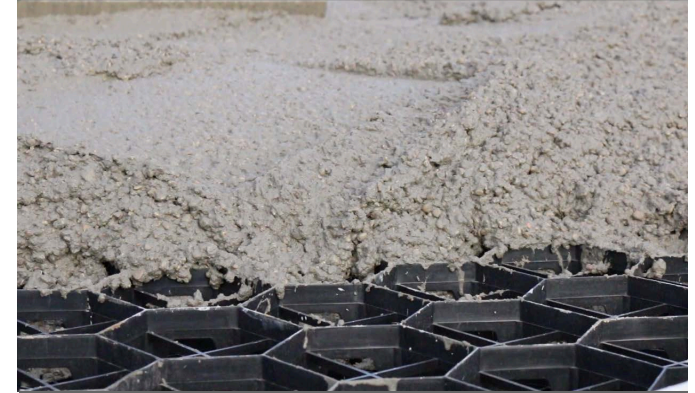
CONCRETE POURING OVER GRID
