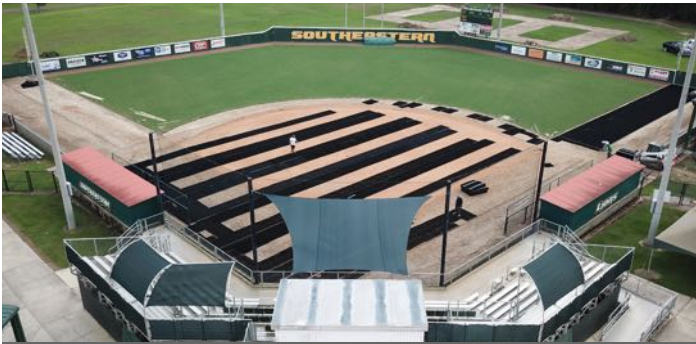
PLACEMENT OF STRUCTURAL GRID
