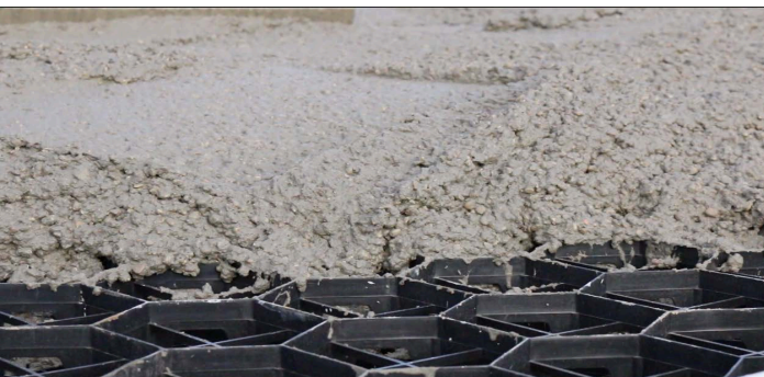
CONCRETE POURING OVER GRID
