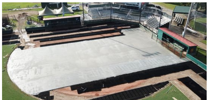
READY TO INSTALL TURF AFTER DRYING
